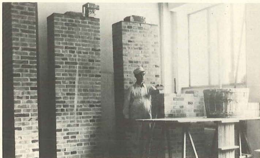
Fig. 8. Opmuring og lagring af mure. Laying and setting of walls.
